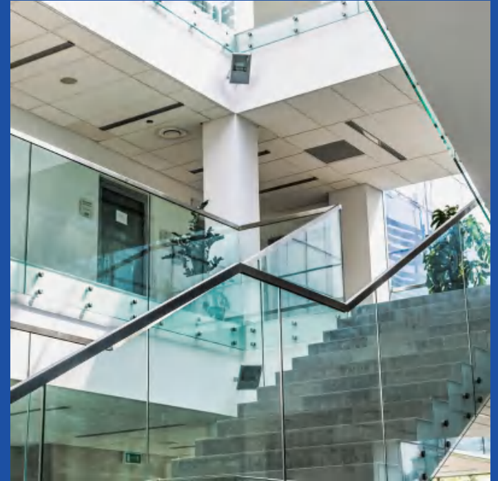
Partrition Support Handrail + PVB Laminated Glass
